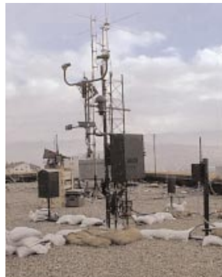
Figure 3-DOD-10. Automated observing equipment deployed to Kosovo.
